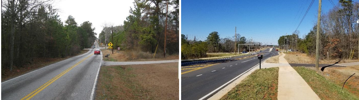
Figure 7-2: Before and After the Anvil Block Road Improvements at Bouldercrest Road
